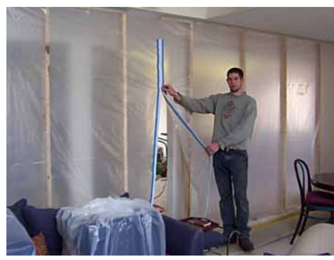
Dust control measures are an important part of protecting your home
