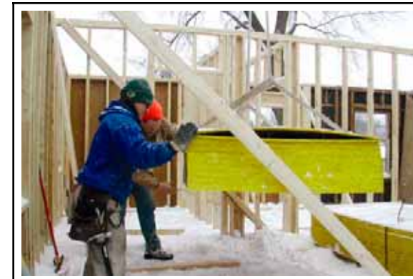
The Heritage crew hard at work on another great remodeling project.
